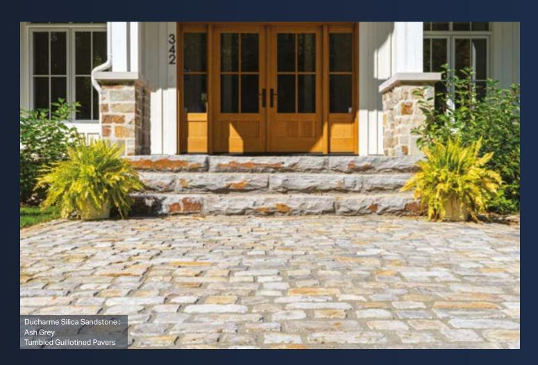
Pavers are guillotined to the desired dimensions and can then be tumbled to give a more natural finish to rounded edges and corners.
